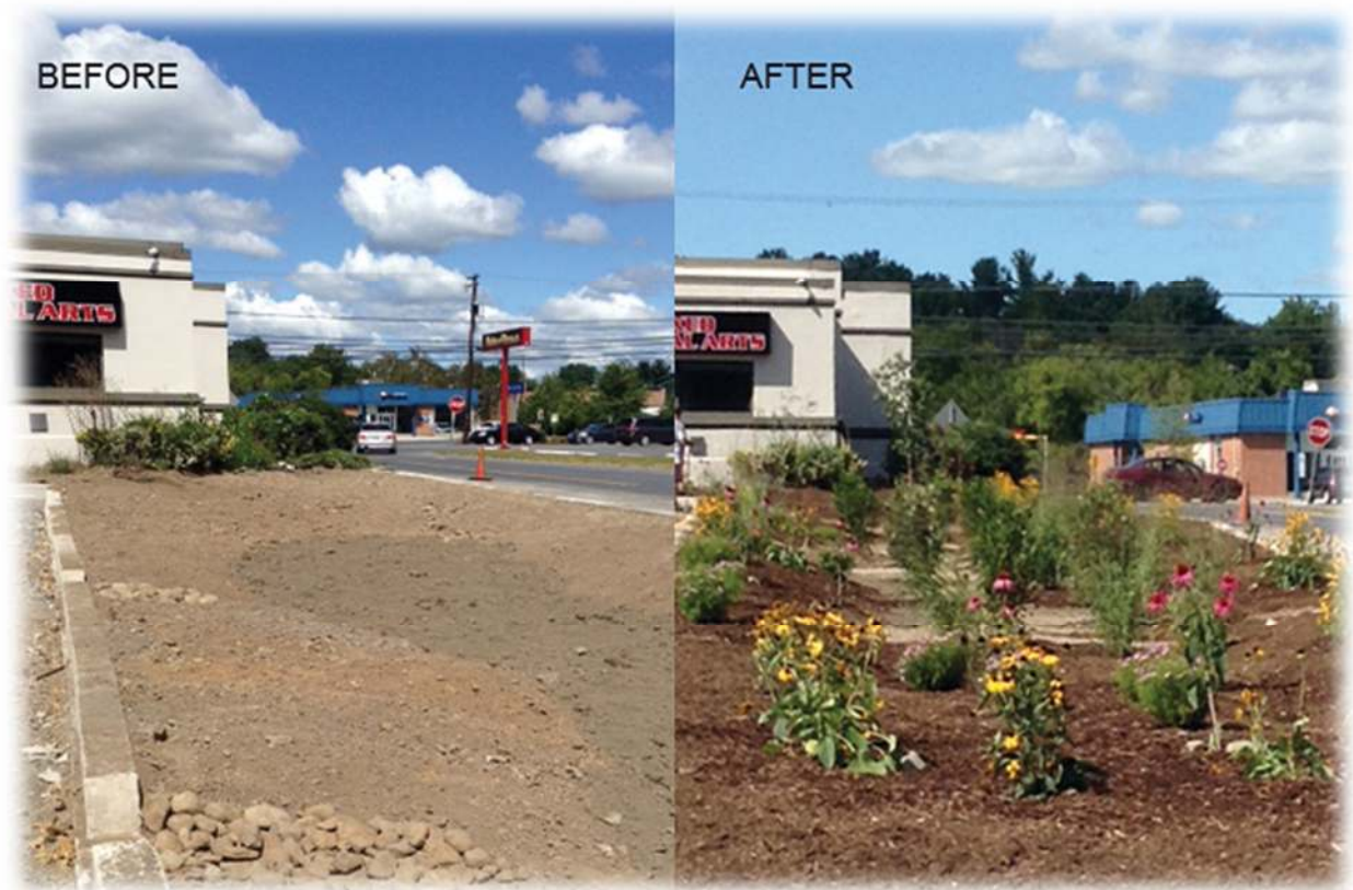
Figure 8: Before and after photos of the installed rain garden at Retro Fitness in Stroud Township.
