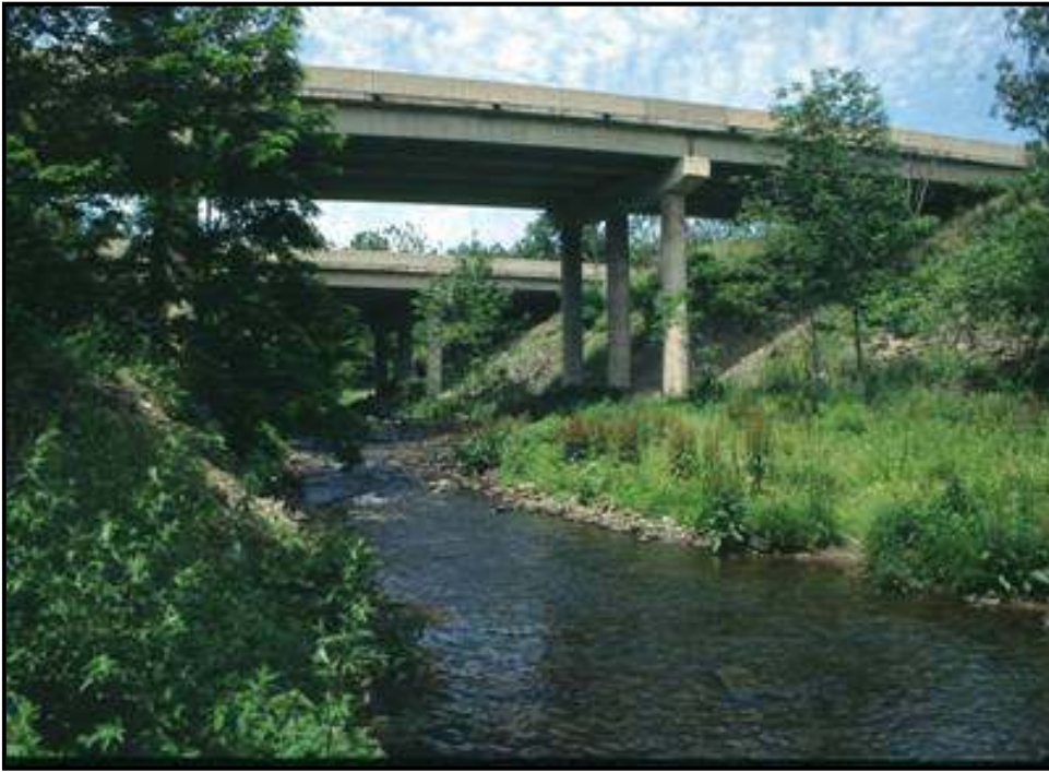
Figure 2.8: Route 80 overpass along the Pocono Creek. (Bob Limbeck, DRBC)
