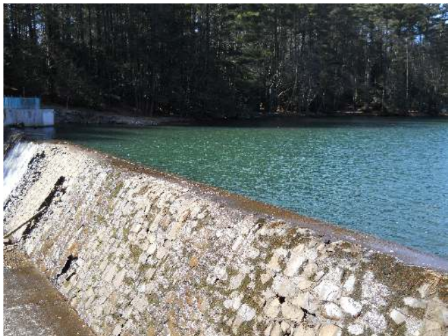
Crawford Lake Dam on the Paradise Creek
