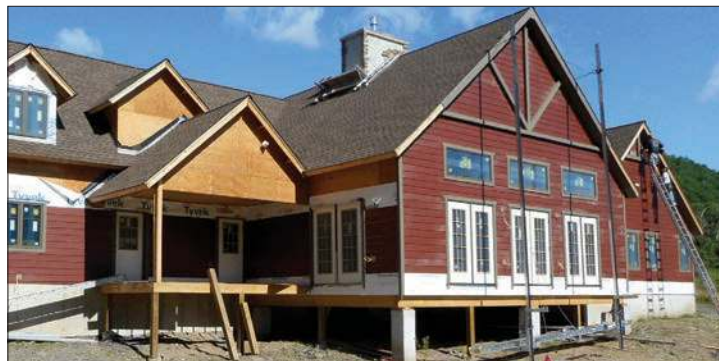
Brodhead Creek Heritage Center will include a large back porch.
