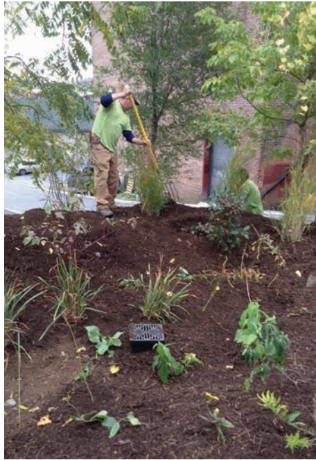
As part of the Green Infrastructure Project, rain gardens were planted at Sarah Street Grill (Quaker Alley, Stroudsburg, pictured here) and at East Stroudsburg High School South. The gardens catch contaminated rainwater from nearby roofs and paved areas, sustaining the native plants and preventing the polluted runoff from reaching the watershed.
